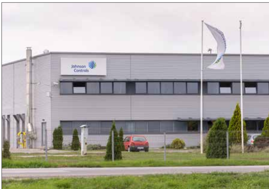
Firma Johnson Controls
